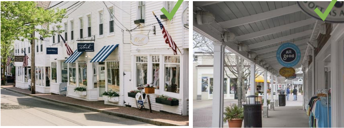
Figure 41 and 42: Example of consistent sign sizes in multi-tenant building Source: visitedgartown.org/shopping and Capecod.com/Mashpee Commons
