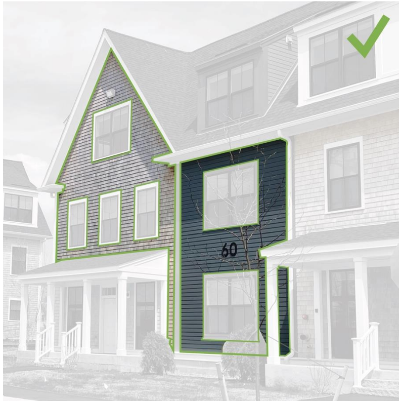
Figure 15: Example of a facade that uses only two materials, including cedar shakes
