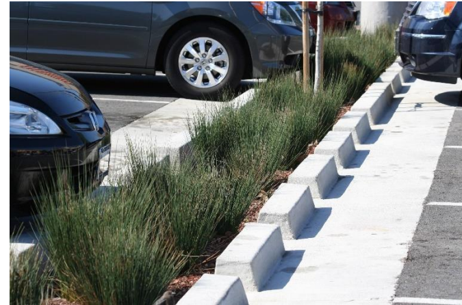
Figure 23: Example of attractive landscape design in parking lot
