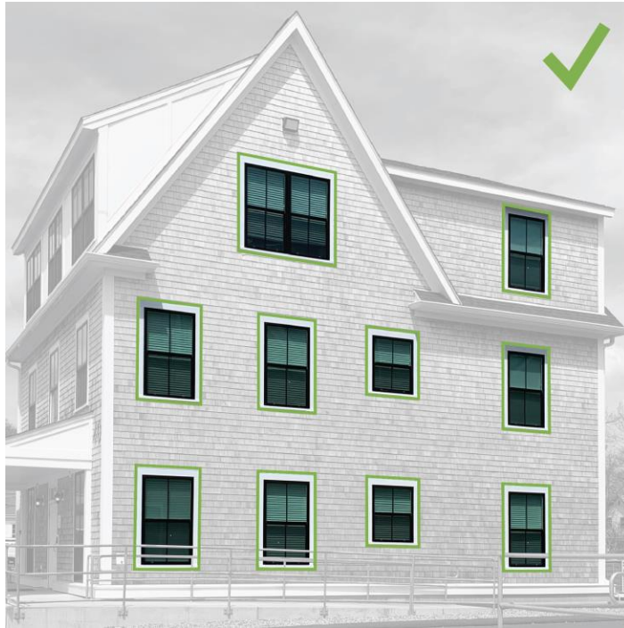
Figure 17: Example of two-over-two sash windows with an exterior muntin
